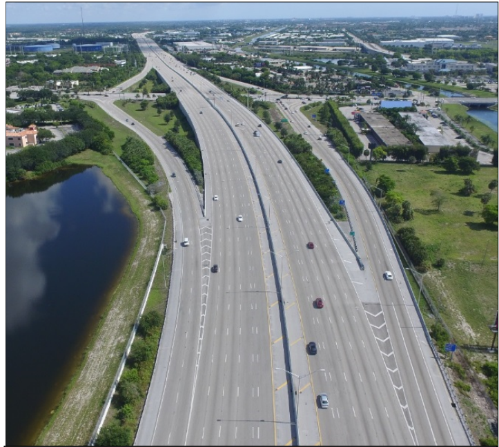
Figure 1-1 I-95 looking north just south of 45 th Street.
